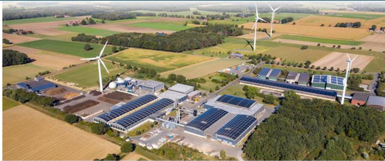
Gescher bio-waste treatment facility (EGW, n.d.)
