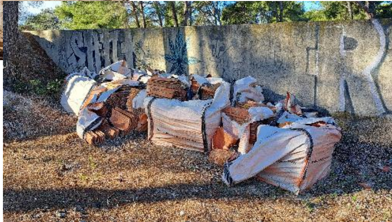
Tiles laid for gabion filling
