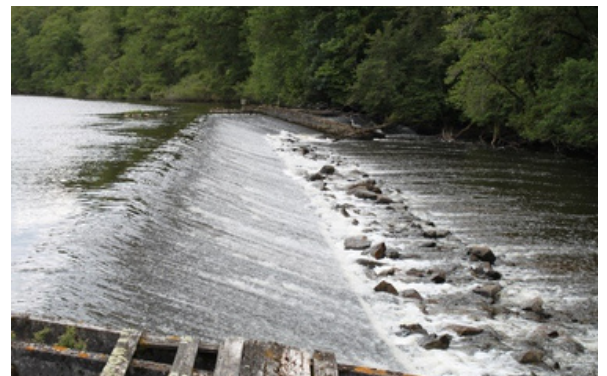
2. THE WEIR AT BEAUFORT
