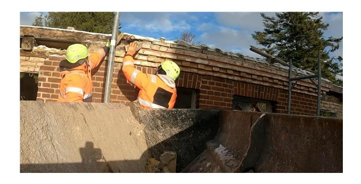
Each brick is cleaned by hand and residues of mortar are removed manually.
