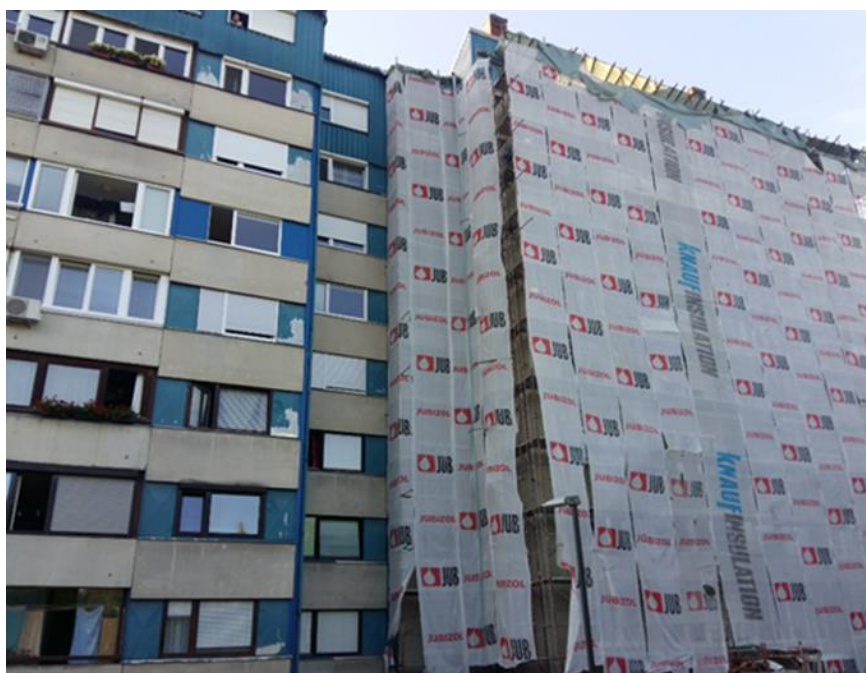
Figure 2: Example of the energy rehabilitation of one part of multi-apartment building
